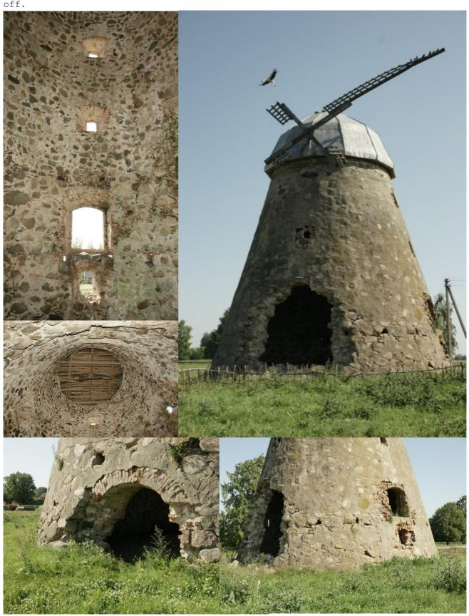
Built in 1905. According to Alis this mill had in the past a fan wheel. Entrance door is not original. Wall are made according to an old building technique. Outside strips are vertical and the wooden strips underneath are laid horizontal.
