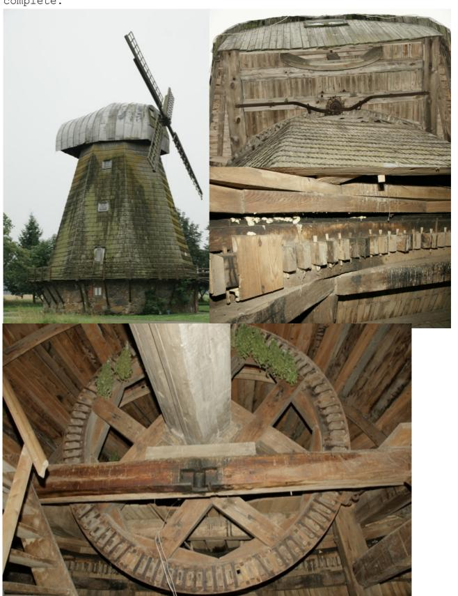
Mill 49, 50 and 51 are at the same location. A lot of mill parts were located aside the windmill. They should have been used for rebuilding the windmill which did not happen. After some years they will be destroyed by sun, rain and wind. Inside the windmill the restoration is to modern. Only the wind shaft itself is old and some parts at ground level inside the windmill.
